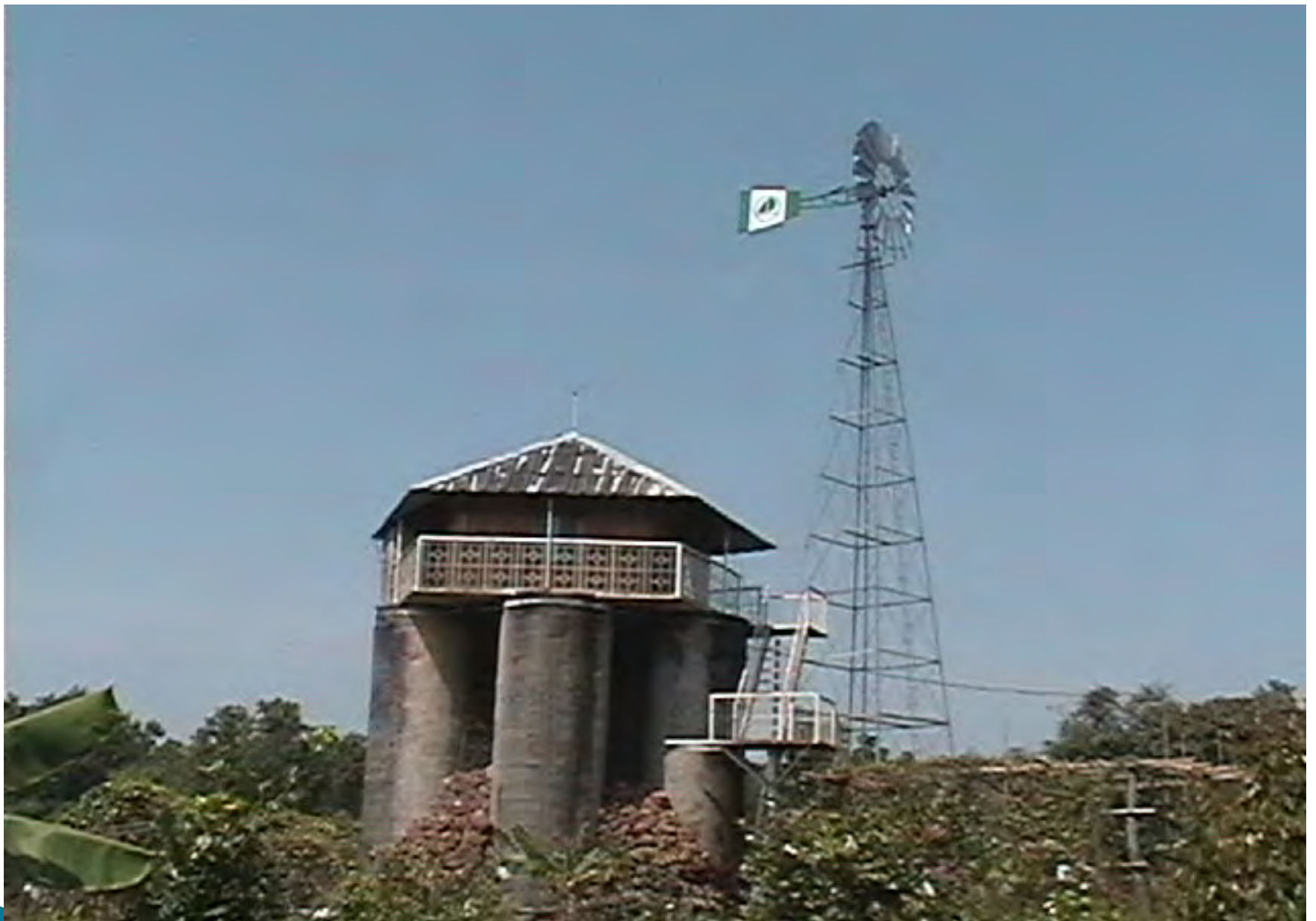
The multi-blade Wind Turbine for water-pumping has been constructed in a farm in Bago Division, Myanmar.
